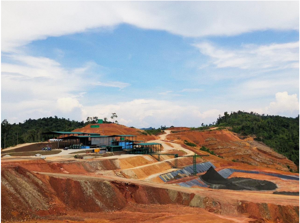
Photo : CIL Plant at Sokor gold field, Kelantan.
